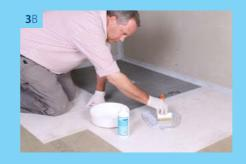
Over-board timber floors using **No**More**Ply** to create a strong, waterproof foundation. Slim 6mm boards fit directly into the tray's rebate. Secure using Mega Strength adhesive and screws.
