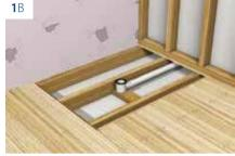
Step 1 Cut out floor boards to the size of the shower tray. Put the trap and waste into position and support with timber to the correct height. The black rubber seal of the trap should be 22mm below existing
